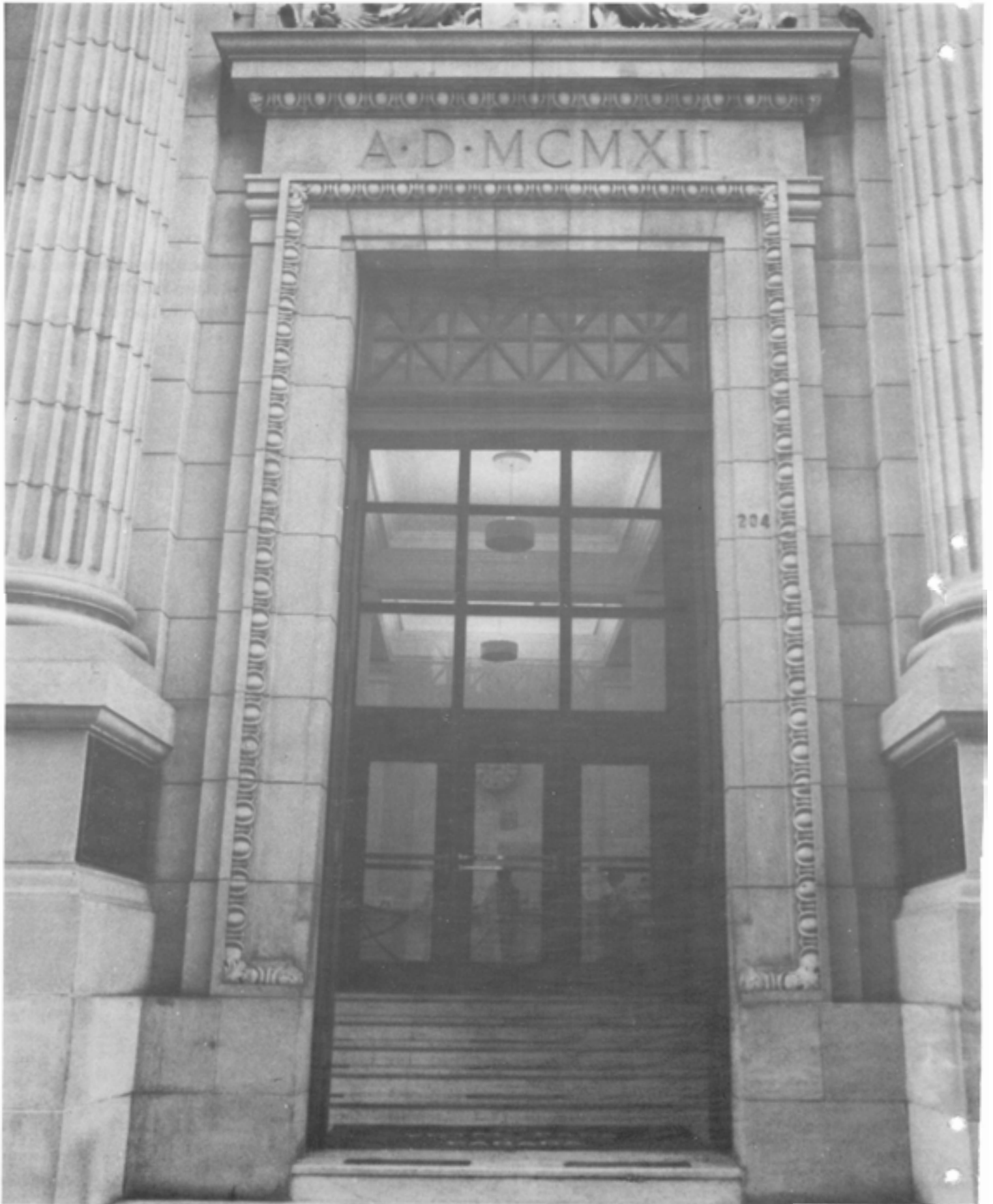
The Royal Bank of Canada - Entrada principal
